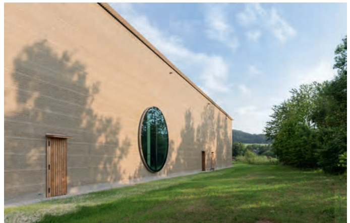
9 Herzog & de Meuron, Ricola Herb Centre, Laufen, Switzerland, 2014 An exterior photograph of the rammed earth building facade.
