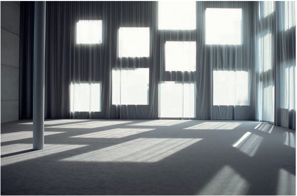
13 SANAA and Heinrich Böll Architekt, Zollverein School of Management and Design, Essen, Germany, 2006 Interior view of facade with closed interior solar and glare protection curtain, highly reflective towards the outside and with a low-e coating towards the space to minimise heat radiation from the hot curtain but reflect the cold activated ceiling.
